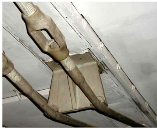
Wood truss c. 1910 with 2-2 1/4" tensioned rods supporting 2 nd floor of car dealership.
