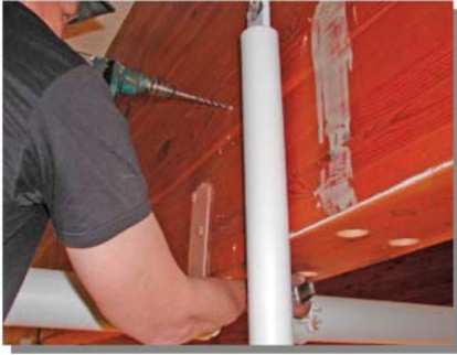
Drilling injection & exhaust ports
