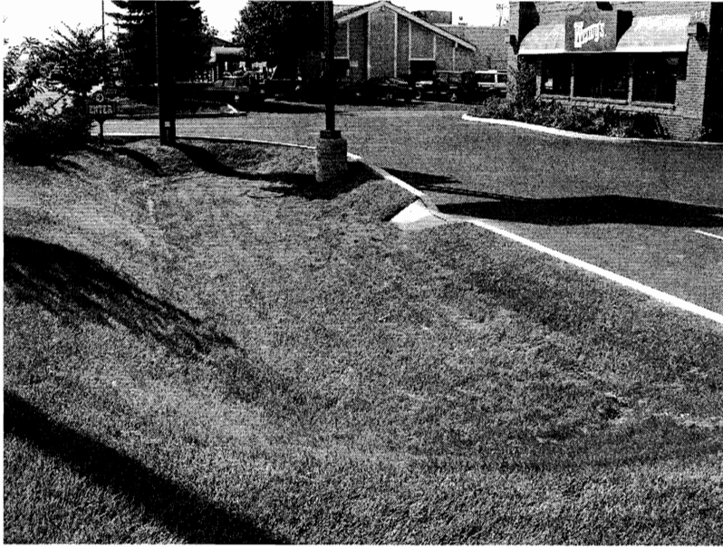
Parking Lot Pond
