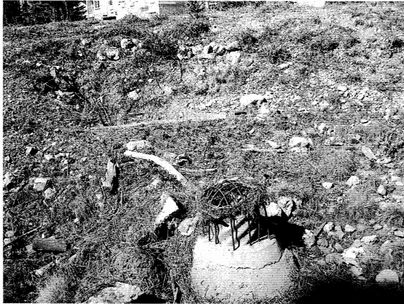
Small Outlet - maintenance
