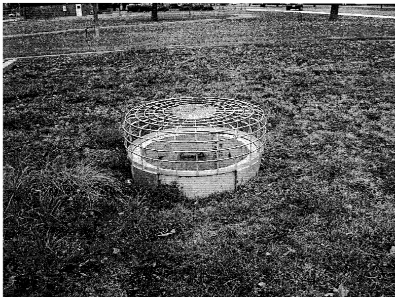
Pond Inlet Structure
