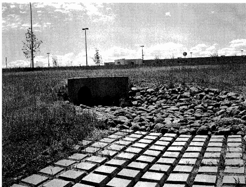
Pond with low-flow channel
