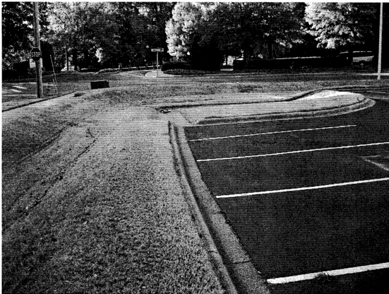
Outlet capacity - grate
