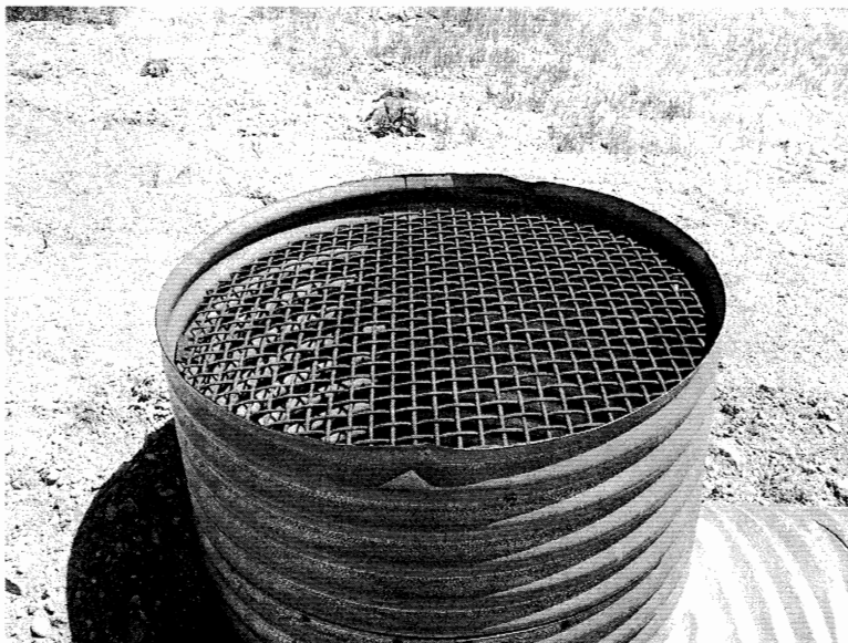
Outlet capacity - Overflow
