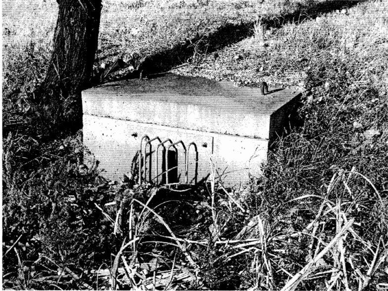
Outlet capacity - concrete structure
