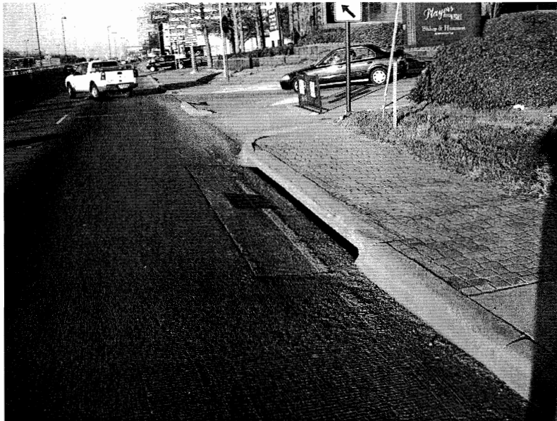
Inlet Types - Curb opening
